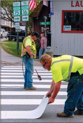
Andrew Whitcomb (left) and Travis Tombley (right) of L & S Property Holdings Inc.'s lay out Hardwick's new thematic crosswalks at the intersection of Main and Hill. The new crosswalks should be more durable than earlier crosswalks. Tombley said that while the new crosswalks are slightly colored on the pavement, summer traffic should shape them to the road so snowplows don't carve them.
