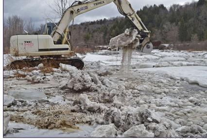
Gary Bellevance of Bellevance Constructors, Inc. opens up a channel at the end of Christian Street in Hardwick, Vermont. The curved pipe cut at the water back to the Cottage Street Bridge so the water could flow more freely.
