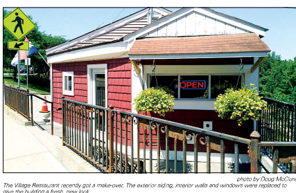
The Village Restaurant, newly open, got a make-over. The exterior siding, interior walls and windows were replaced to give the building a fresh, new look.
