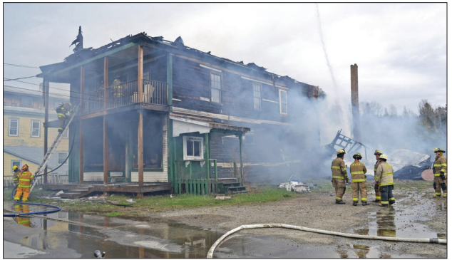
Thick smoke filled the air Friday as eight fire departments put out a fire that started in an empty multi-unit apartment building on Main Street in Greensboro Bend. The building has been empty for several years and is owned by Michael Goldberg of Alameda, California.
